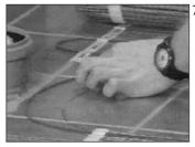
If required, the cable can be removed from the mesh and loops formed manually, but ensure the cables are spaced the same distance as those on the mat.
