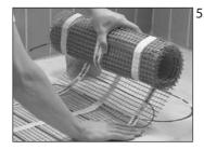
Before laying the mat should be tested-see page 7. Remove the plastic outer and place the cold tail of the mat at the connection point. The Devimat<sup>™</sup> has a self-adhesive backing, lay this to the floor and roll the mat out, if necessary the mat can be laid with the cable face down. In situations where the mat has to be turned over it can be secured using Devipins, hot glue gun (taking care not to damage the heating cable), staple gun or double sided tape.
