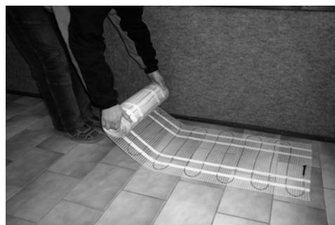
Dry fit the mats
