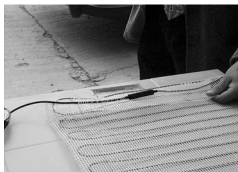
Cut a channel for the power leads
